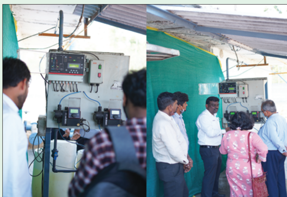
CLO 2 treatment system for odour control in operation in RCF based paper mill.
